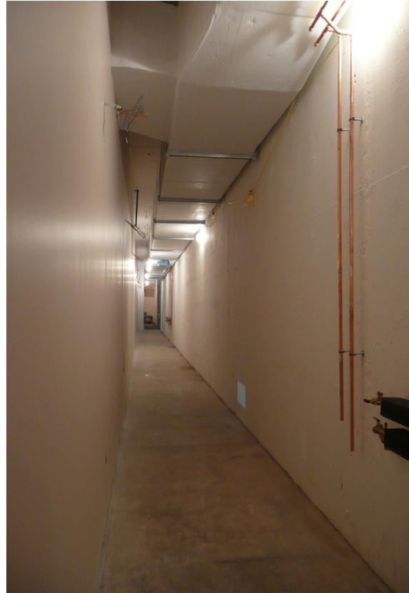
**FIGURE 11.7.** Typical buffer space between conditioned space and exterior wall (right of image).
